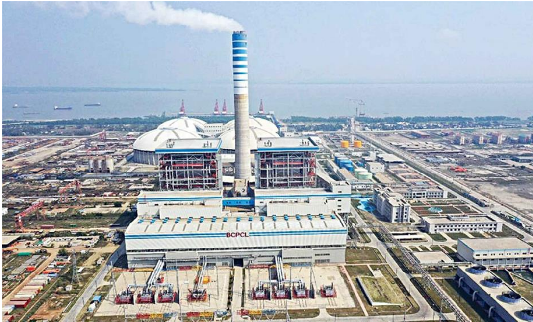
Figure 12-5: A View of the 1320MW Coal-Fired Power Plant in the Dhankhali Area
